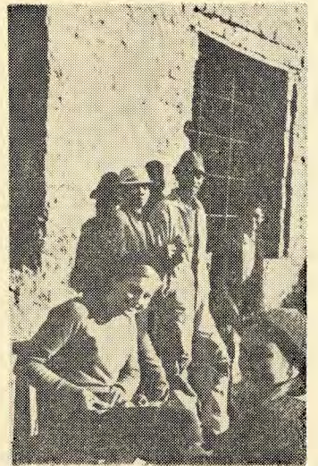
Job reservation at the Shiloh workcamp? Women were delegated to soften putty and glaze window panes. Eleven windows were put into the three foot thick walls.
