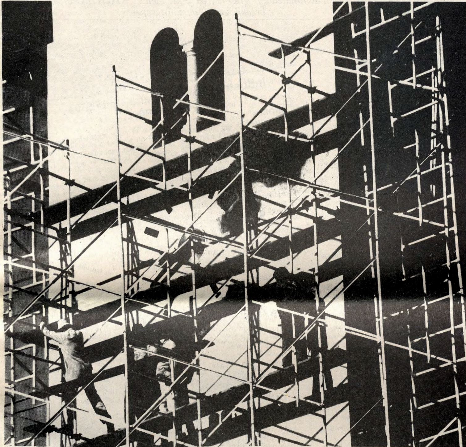
As admin tries to hide the cracks, the ivory tower crumbles.
